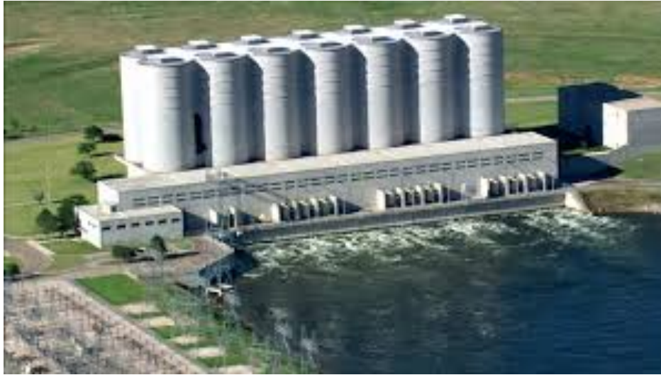
Oahe Dam Powerhouse near Pierre, SD – Note the Oahe Irrigation Pumphouse to the right. Construction on the facility had started before being halted in the late 1970s
