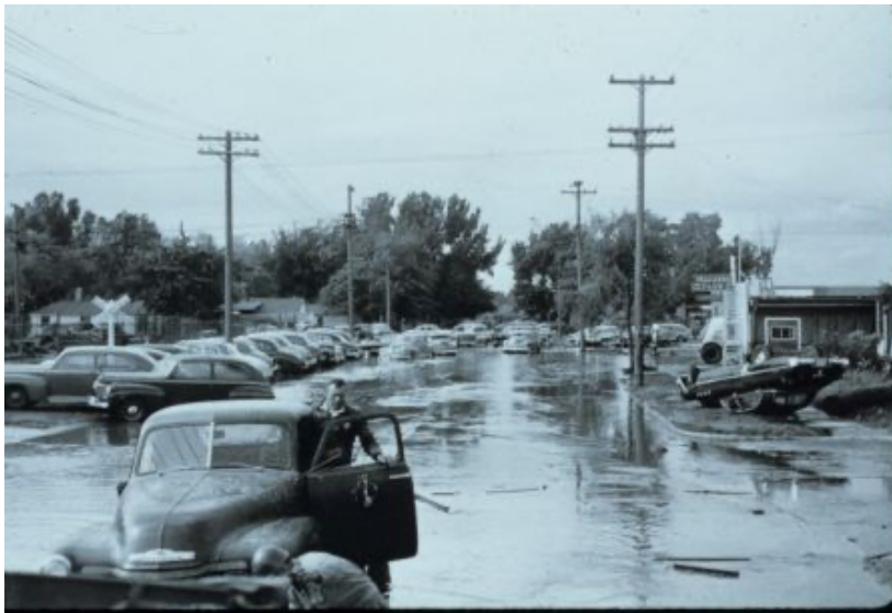
Flooding on the Missouri River Circa 1943
